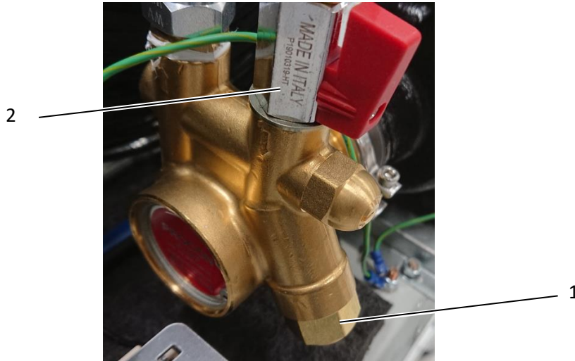
Fig. 11: Locations of ball valve and strainer
